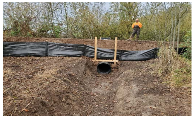
Water control structure post-installation
