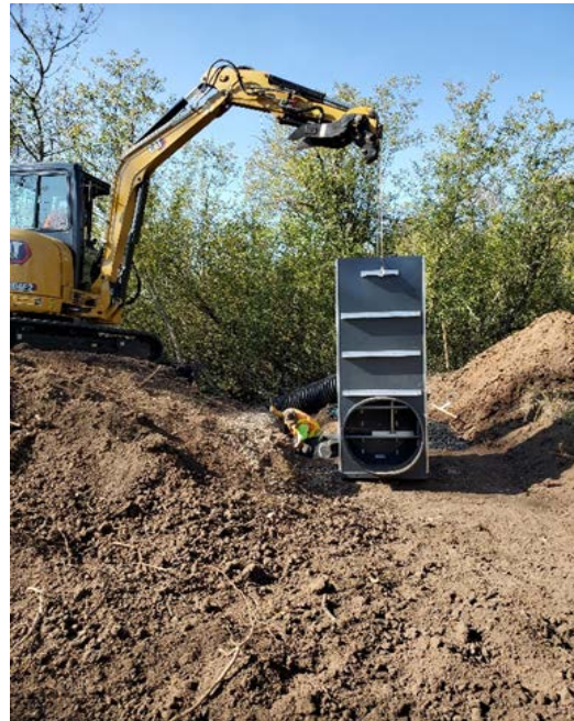
Water control structure being installed at Fern Ridge Wildlife Area.
